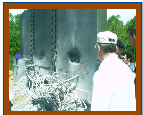
Image 2 - Damage to concrete bolsters
