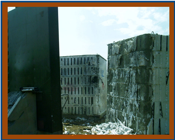
Image 4 - Blast area on May 8, 2003
