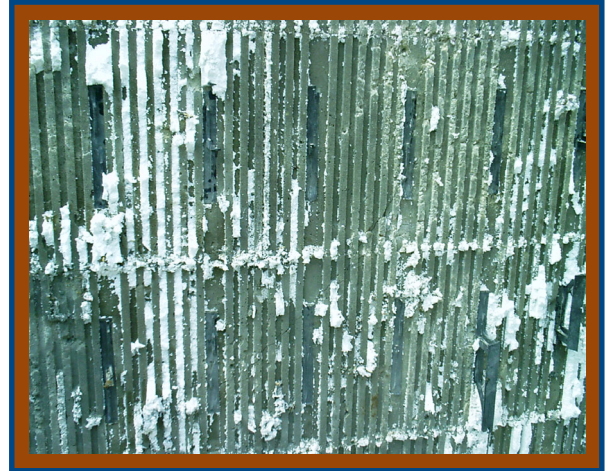
Image 5 - ICF wall at six feet
